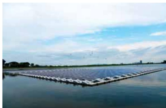
**Figure 1. Ciel et Terre's floating solar mount is an example of the pure-float design**
