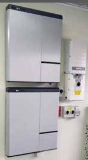
**DC coupling residential solar and batteries results in more energy production and increased return on investment, according to SolarEdge**
