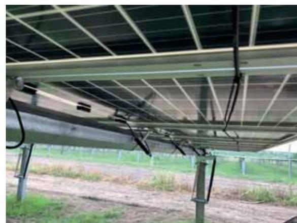
**Figure 1. Wiring considerations for bifacial modules: to prevent shading of the rear-side of the module how the DC wire harnesses will travel down the racking structure without shading the rear side of the modules must be considered during the design and procurement stages of the project. Different modules paired with different racking structures require custom approaches**
