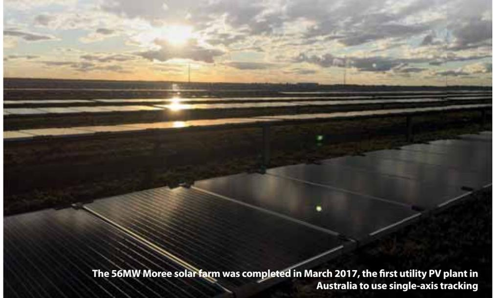
The 56MW Moree solar farm was completed in March 2017, the first utility PV plant in Australia to use single-axis tracking
